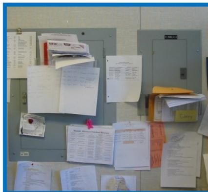
Decorative materials or paper must not be placed on EXIT doors, in exit stairwells, over fire alarms, over electrical panels, outlets or switches.
